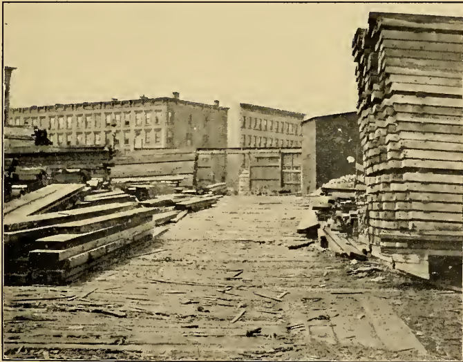
COURSE OF CHURCH LANE AS IT IS TO-DAY. VIEWED FROM VERVEELEN'S FERRY SITE AT 125TH STREET AND HARLEM RIVER.
